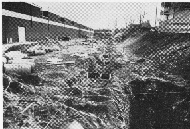
MILL ADDITION PROCEEDING ON SCHEDULE. Concrete footings are being poured (left) for the new 62,000-foot mill addition in the Waterbury East Plant. Right: as sketched by the architect, the new building is being added
